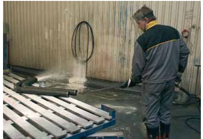
The prefabricated piping modules are then washed with 110°C–130°C steam (to which a chemical cleaning agent has been added).
