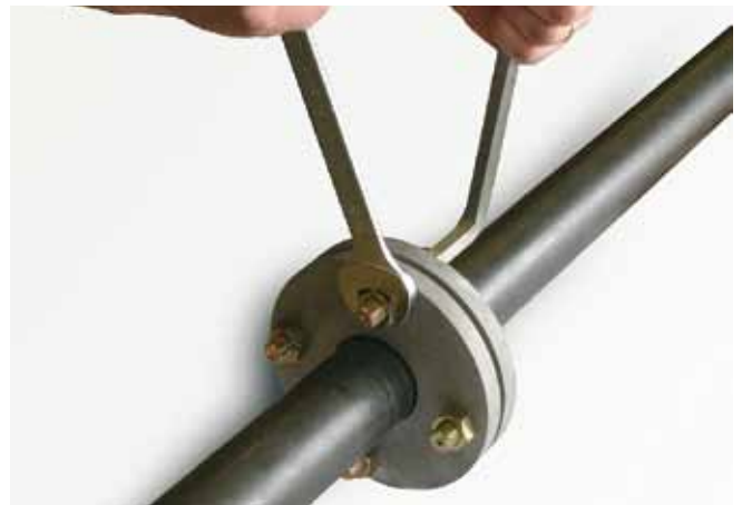
The greased bolts (and nut) are tightened to the given torque to complete the installation.
