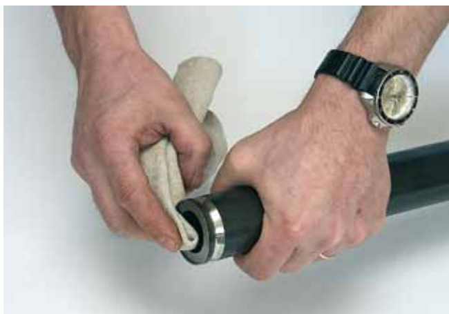
The cover is removed from pipe end and the pipe is cleaned with a doth.
